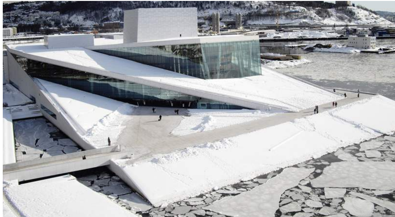
Snohetta Oslo Opera House - Large Stone & Marble Slabs
